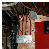
SMOKE AND FIRE ALARM : CHURCH AFTER INSTALL
